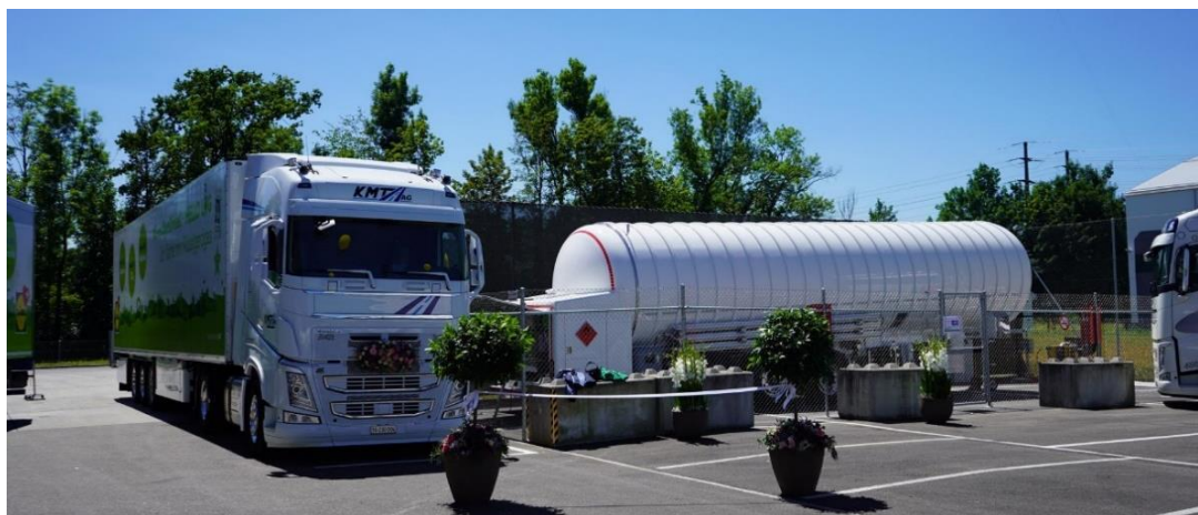
Fig. 6. LNG Service Station in Weinfelden, Switzerland
