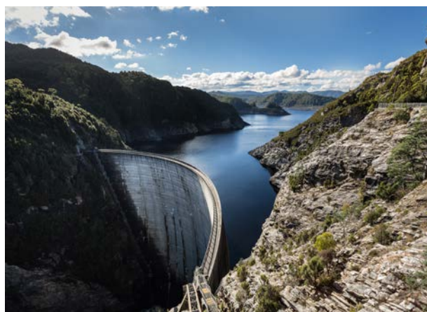
Gordon Dam in Tasmania (Photo courtesy of Hydro Tasmania)
