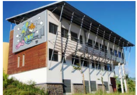
ENERPOS, a net zero energy building in Reunion Island, a tropical climate. (Photo courtesy of Francois Garde)
