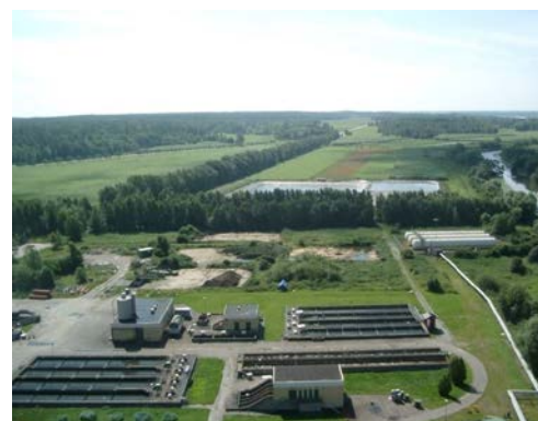
Municipal wastewater plant in Enköping, Sweden, with water storage ponds and (behind the ponds) willow fields that are used as vegetation filters, the harvested willow fuelling an adjacent power plant - (Photo: Pär Aronsson, SLU)
