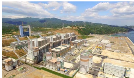
The new 4x550 MWe FBC combustor in Samcheok, South Korea (courtesy of KEPCO, 2019)
