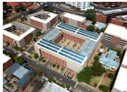
Wits Junction solar system is the largest solar thermal installation in Sub-Saharan Africa. It combines solar, co-generation and gas heating technologies, servicing 14 student residence buildings with one centralised hot water plant. Installation includes a 600m 2 heating plant with 10m 2 of collectors. (Source: Wits Junction/SOLTRAIN).
